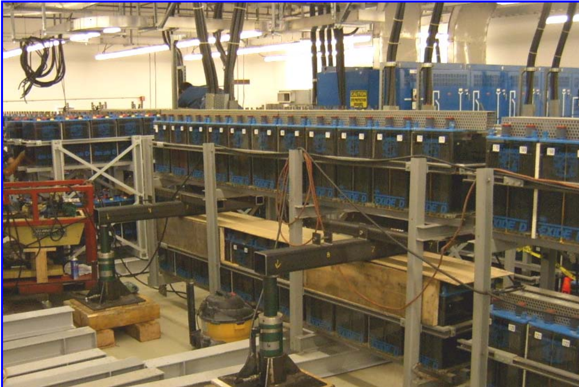
Fig 1. A very unique project, this client required massive above slab reinforcement to accommodate the weight of a flooded battery addition to its existing UPS battery room.
