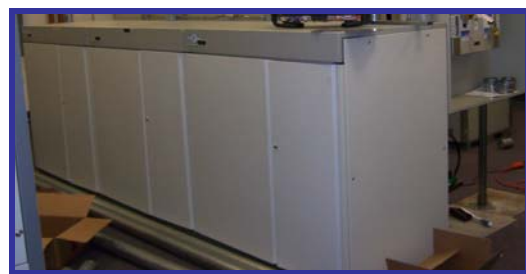
10 yr VRLA batteries in cabinets
