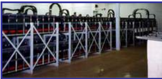
Fig. 2a, b 20 yr Flooded batteries/racks
