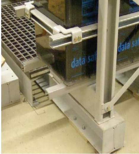
Addition of grating
